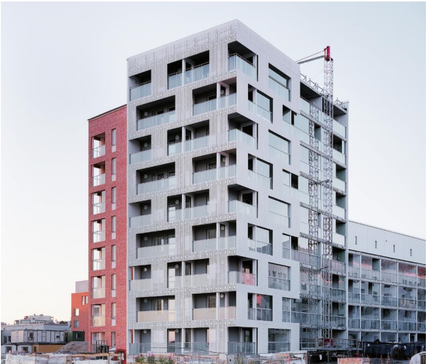
550 m² fibreC 3D elements with a thickness of 7 cm are cladding the Lontoonkatu 9 project in Helsinki, designed by Kirsi Korhonen and Mika Penttinen Architects. The entire facade was divided into 16 different types of panels with lenghts up to 3.8 m. More than 400 concrete elements with faced concrete quality on both sides offer an interesting view from inside of the building.
